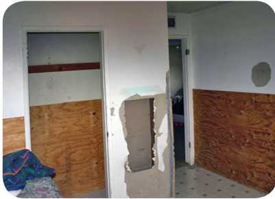
Holes in walls
