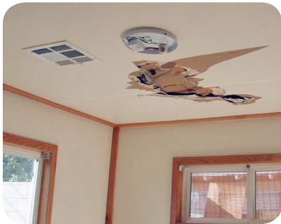
Holes in ceilings
