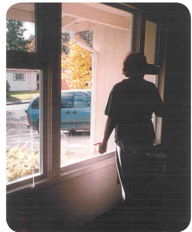
Plexiglas sheet installed to protect the living room window
